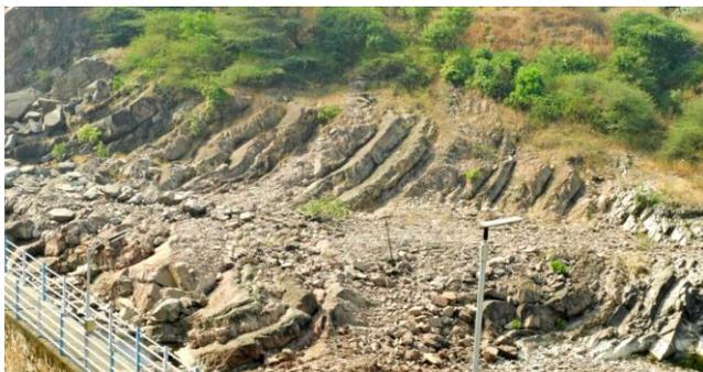
**Erosion on Downstream side due to Overflow of water from Spillway Section**
