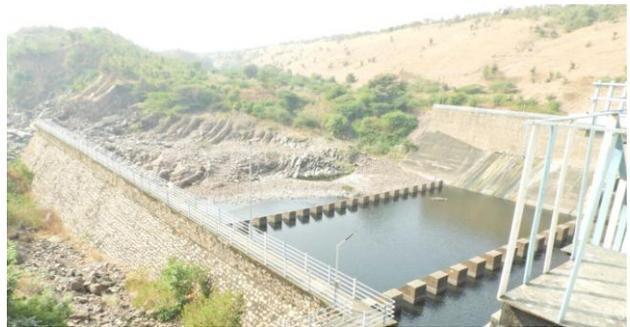
**Downstream side of Watrak Dam with Energy Dissipators**
