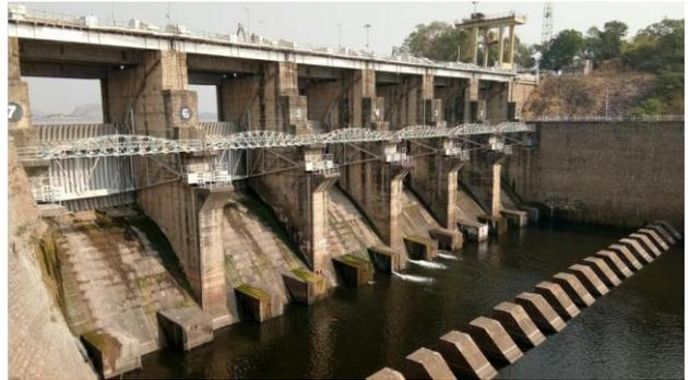
**Ogee type Spillway at Watrak Dam**
