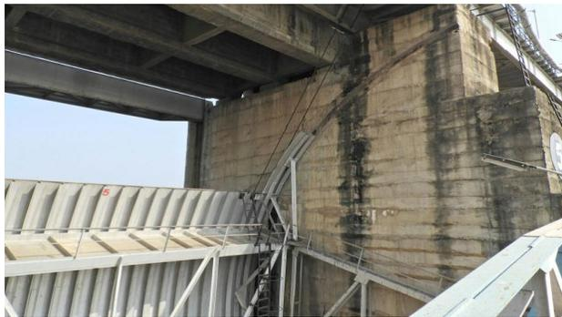
**Radial Gates of Ogee type Spillway at Watrak Dam**
