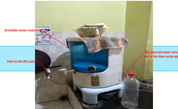
Figure 5: RO System installed in home
